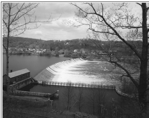
Left: The Derby Dam, constructed in 1870 bordering Shelton and Derby, was the first hydropower dam on the Housatonic River. Huge ice floes burst the dam in 1890 and it was reconstructed. Now, it is no longer used.
